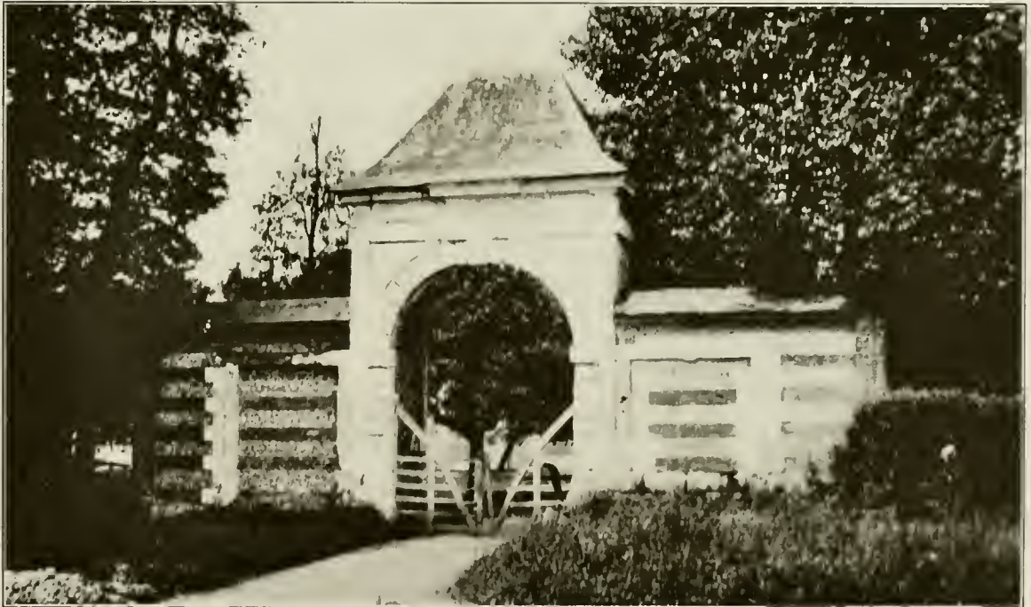
PLATE 179. Farm entrance near Lintot, Seine-Inférieure
